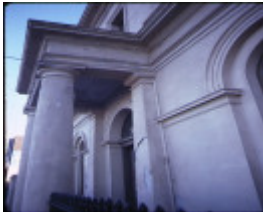
former es&a bank clunes front columns
