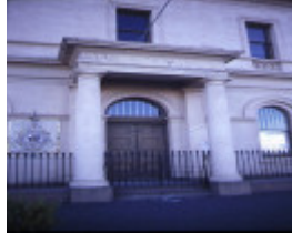
1 former es&a bank clunes front entrance
