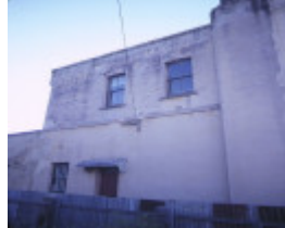
former es&a bank clunes back windows
