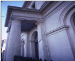
former es&a bank clunes front columns
