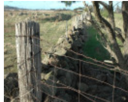
Dry Stone Wall R193
