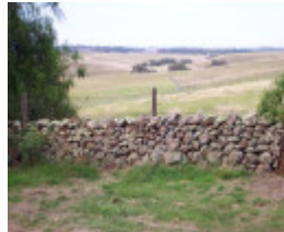
Dry Stone Wall R6
