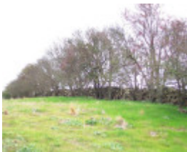
Dry Stone Wall R6
