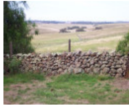
Dry Stone Wall R6
