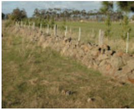
Dry Stone Wall R193
