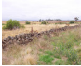
Dry Stone Wall P298
