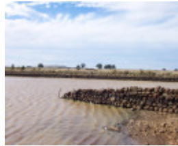
Former Clarke Dam
