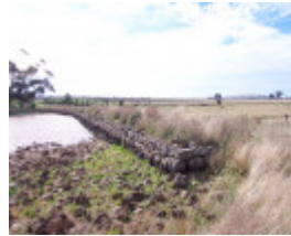
Former Clarke Dam
