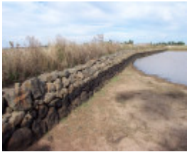
Former Clarke Dam
