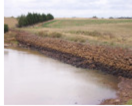
Holden Road Dam
