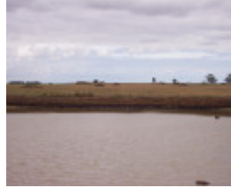
Holden Road Dam
