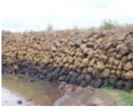
Holden Road Dam
