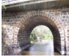
Bridge over the Kororoit Creek
