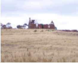
Mount Aitken site and ruin
