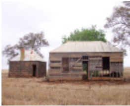
Bluestone cottage and timber dwelling
