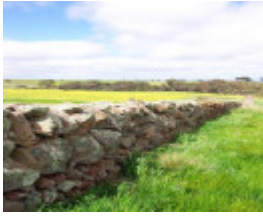
Dry Stone Wall A274
