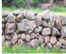
Dry Stone Wall A276
