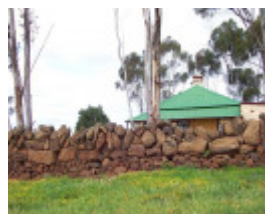
Dry Stone Wall A272
