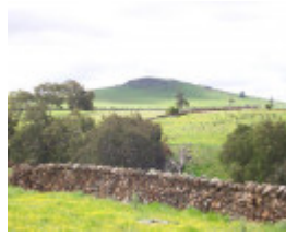
Dry Stone Wall A275
