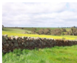
Dry Stone Wall A274
