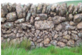
Dry Stone Wall A277
