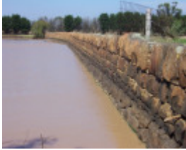
The Plumpton Dam
