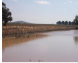
The Plumpton Dam
