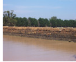
The Plumpton Dam
