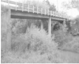
Bridge Road bridge over the Toolern Creek
