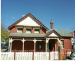
Former Melton Courthouse
