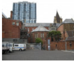
Francis Ormond Bldg_Melbourne_rear view_8 Jan 2008
