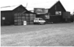
Towts Cool Store & Packing Shed
