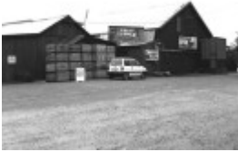
Towts Cool Store & Packing Shed
