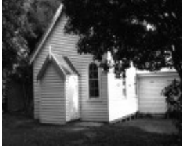
Tynong North Methodist Church - Former Christ Church
