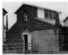
Warrawong Shearing Shed
