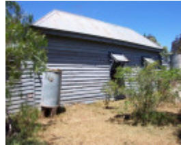
Side elevation of farm house
