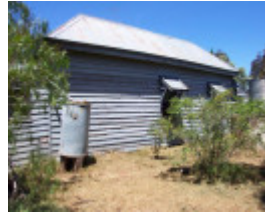
Side elevation of farm house
