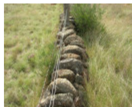
Dry Stone Wall K164 - Eastern Boundary
