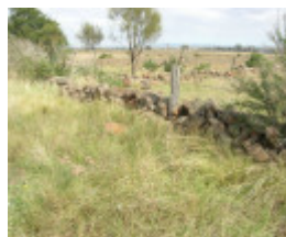
Dry Stone Wall K164 - Eastern Boundary
