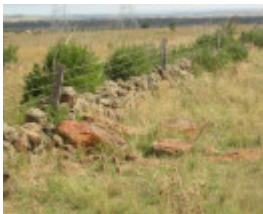
Dry Stone Wall K165 - north boundary
