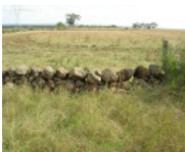
Dry Stone Wall K164 - Eastern Boundary
