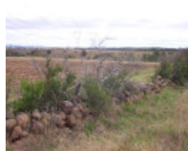
Dry Stone Wall K165 - north boundary
