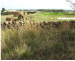
Dry Stone Wall K159 - eastern boundary
