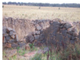
The ruins of the rubble bluestone house
