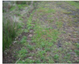
Rockbank Middle Road pavement
