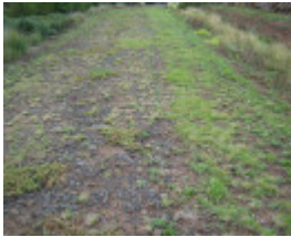
Rockbank Middle Road pavement
