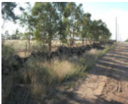
Dry Stone Wall F186 - southern boundary
