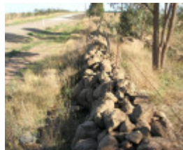
Dry Stone Wall F186 - southern boundary
