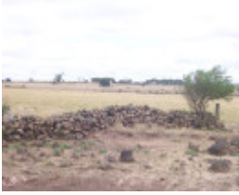
Dry Stone Wall F19 - walls in centre of paddock
