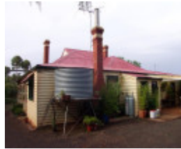
Rear elevation of house
