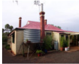
Rear elevation of house
