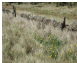
Dry Stone Wall B76
