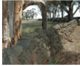
Dry Stone Wall B75
