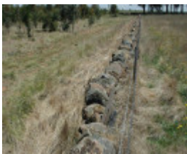
Dry Stone Wall B76
