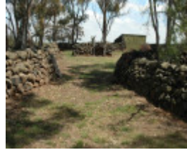
Dry Stone Wall B75
