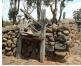
Dry Stone Wall B75
