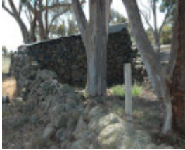
Dry Stone Wall B75
