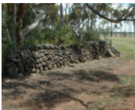
Dry Stone Wall B28
