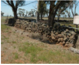
Dry Stone Wall B74
