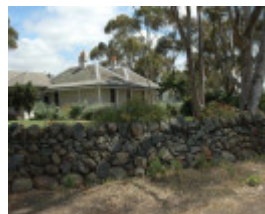
Dry Stone Wall B28
