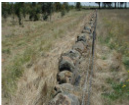
Dry Stone Wall B76
