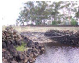
Dry stone wall dam, with cobbled ramp
