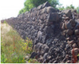
Rockbank Headstation Dam Wall
