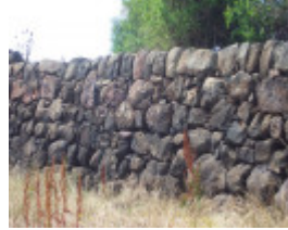
Rockbank Headstation Dam Wall
