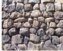
Rockbank Headstation Dam Wall - detail
