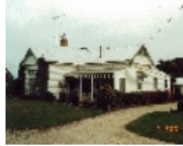
Dwelling at 5967 South Gippsland Highway
