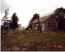
Arawata State School No. 2970 (former)
