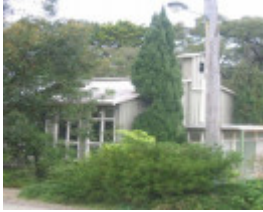
Maryknoll Residential & Civic Precinct - Residence
