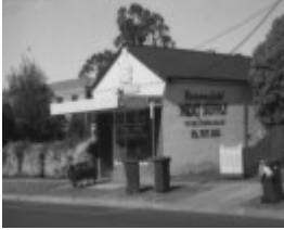
Wood Street Commercial & Civic Precinct
