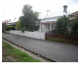
HO7(2) - Old Footscray Township Residential Area.JPG
