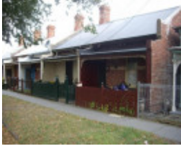
HO7(1) - Old Footscray Township Residential Area.JPG
