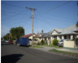
HO12(5) - War Service Homes, Heritage Area, Maribyrnong.JPG
