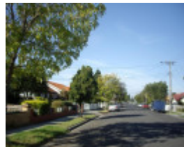
HO12(4) - War Service Homes, Heritage Area, Maribyrnong.JPG
