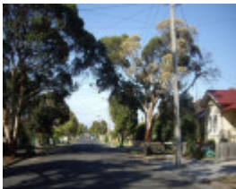
HO12(1) - War Service Homes, Heritage Area, Maribyrnong.JPG
