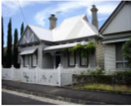
HO13 (2) - William Angliss worker housing estate heritage area, Footscray.JPG
