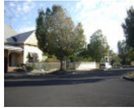
HO13(1) - William Angliss Workers Housing Estate.JPG
