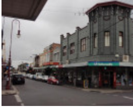
HO14(3) - Yarraville Civic and Commercial Heritage Area.JPG
