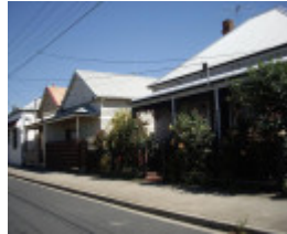
HO15(4) - Yarraville residential heritage area.JPG
