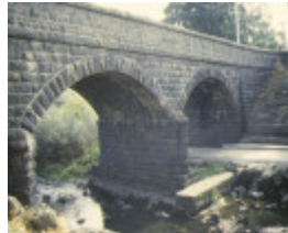
bridge newlands road coburg side detail
