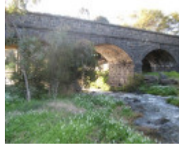
H1446 Newlands Road Bridge 3 Sep 2008
