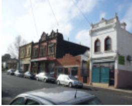
Union Street shops
