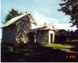
Dollar State School No. 3473 (former)
