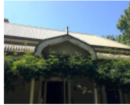
Greenfields verandah gablet
