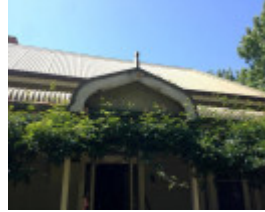
Greenfields verandah gablet
