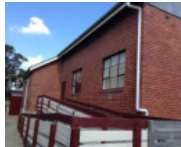
Fish Creek Memorial Hall 1959 Supper Room addition
