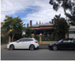
36 Green Street, Windsor
