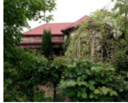
House 23 Bridge Street
