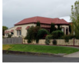
House 23 Bridge Street
