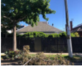
66-72 Peel Street, Windsor
