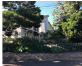
66-72 Peel Street, Windsor
