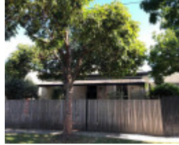
66-72 Peel Street, Windsor
