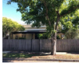
66-72 Peel Street, Windsor
