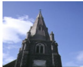
holy trinity anglican church complex sydney road coburg spire detail aug1992
