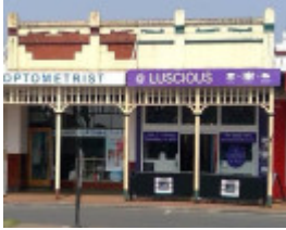
Shops, 7-9 Commercial Street (2020)
