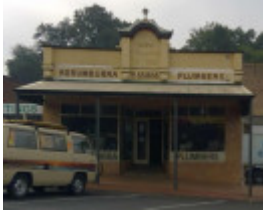
Falconer Building (former, 2020)
