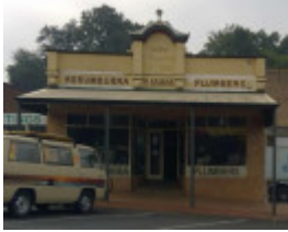
Falconer Building (former, 2020)
