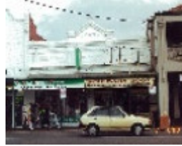
Shops, 8-10 Bair Street (2000)
