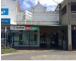
Shops, 8-10 Bair Street (2020)
