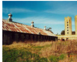
View of south shed and silos
