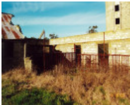
View between milking sheds at rear, near silo
