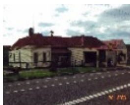
Former Bigelow's Store
