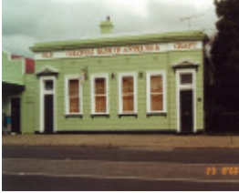
Former Colonial Bank of Australasia
