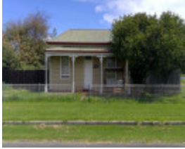
House, 6 Turnbull Street (2020)
