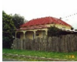
House, 6 Turnbull Street (2000)
