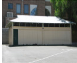
AUBURN PRIMARY SCHOOL NO.2948 SOHE 2008
