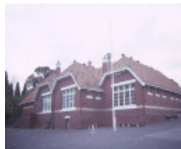
auburn primary school no 2948 rear view
