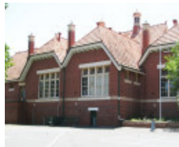
AUBURN PRIMARY SCHOOL NO.2948 SOHE 2008
